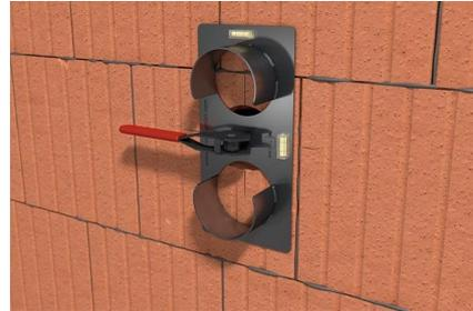
Insert drilling template, fasten with template lever with quick-clamping function and align.
