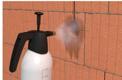
Slightly moisten the can bore, so that thermal foam swells more quickly.
