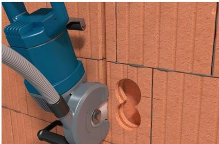
Mill slot with cutter next to holes, additionally mill to just before or into can hole.
