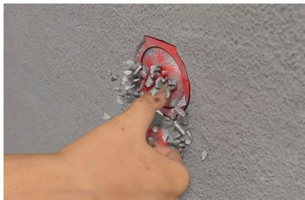
Press in plaster lid by hand, alternatively drill out plaster lid with drill bit.
