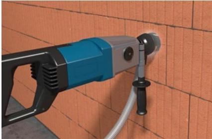
Mark first box and drill out with 82mm drill bit
