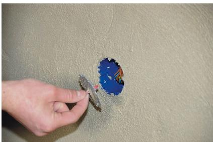
Remove the cleaning spring and mill the can lid with the help of the centering drill hole.
