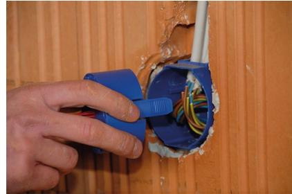
Carefully engage standard lids with interlocking detent teeth.
