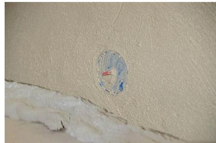
When plastering, the plasterer presses the cover to the required height - flush guaranteed flush with the plaster and VDE-compliant!
