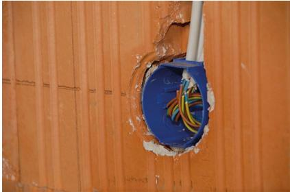
Set bottom part flush, insert cables or insert pipes.
