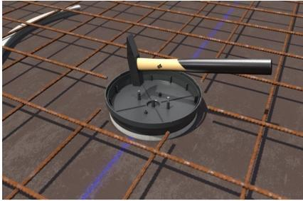
Nail the front part with mineral fiber board to the formwork. The integrated nail fixation in the front part enables easy assembly.
