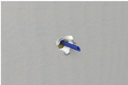
Push beveled mandrel through second plasterboard, if necessary first hammer in hole with hammer.
