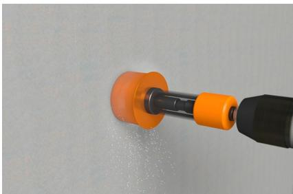
Place the box cutter in the centering hole and mill out the hole.
