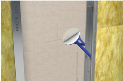
Stick the adhesive disc onto the wall and remove the protective film.
