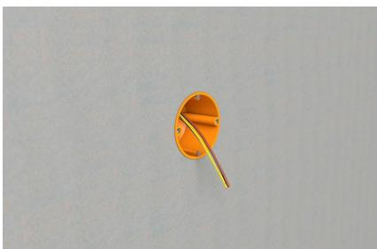
Install cavity wall box, install recessed appliance or socket.
