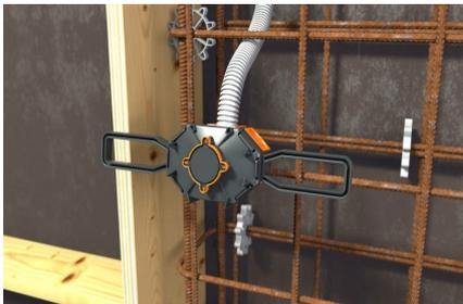
Variant 2: Attach attachable wings to membrane box and fasten to steel reinforcement with wire.
