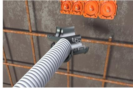
Open manifold and attach M32 installation pipe. Or...
