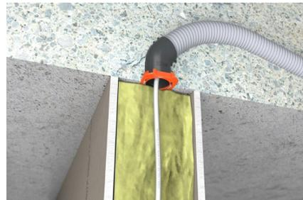
Suitable for installation in lightweight walls and possible continuation of installation pipes.
