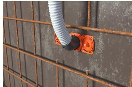
Plug the elbow onto the front part. Ideal bending radius according to DIN.
