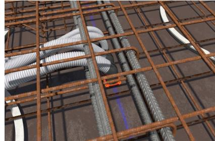
Toolless pipe insertion M32-M40. Plug elbows and grommets onto the front part. Ideal for installation situations with a lot of reinforcement.
