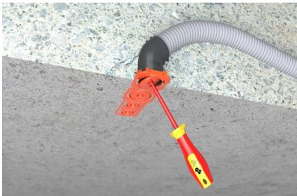
After concreting, the opening can be broken out with a screwdriver.
