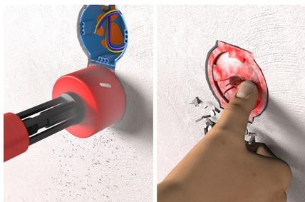
Drill out plaster cover with drill bit or press in by hand.
