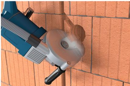
Mill the slot into the can bore using a milling cutter..
