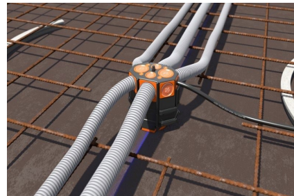
Open the diaphragm with a cutter knife open and insert tubes and cables.
