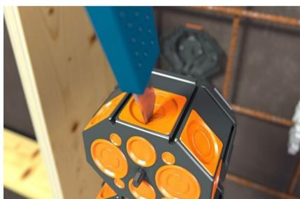
Open the diaphragm with a cutter knife.
