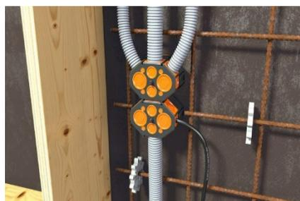
Tool-free insertion of cables and (rigid) pipes.
