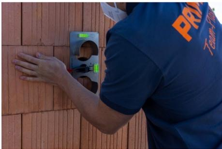
Attach the template lever with the quick-release function.
