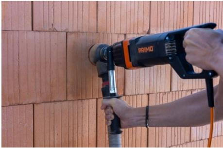
Measure the first hole and mill out with Primo high-speed runner.
