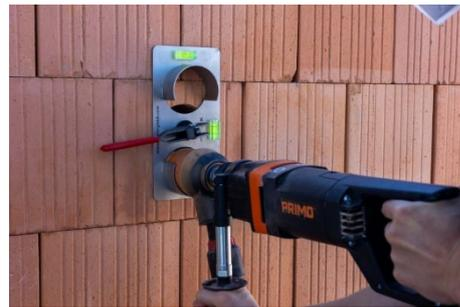
Insert the high-speed runner with a  $\varnothing$  82 mm drill bit straight into the drilling template and mill out further drill holes. No centering drill is required!
