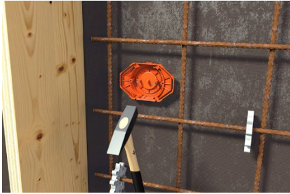
Variant 1: Nailing the front part to the formwork. The integrated nail fixation in the front part enables easy assembly.
