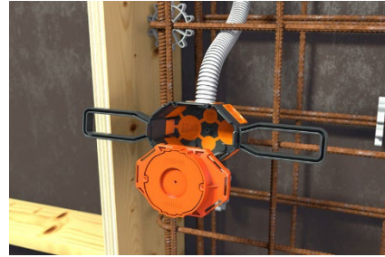
Variant 2: Attach wings to membrane box and attach with wire to steel reinforcement.
