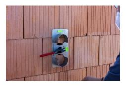
Insert and align the drilling template. Spirit levels ensure precise installation.
