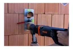
Insert the high-speed runner with a Ø 82 mm drill bit straight into the drilling template and mill out further drill holes. No centering drill is required!
