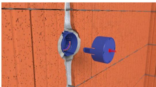
Snap the upper section into the lower section so that it protrudes by approx. 2.5 to 3 cm.
