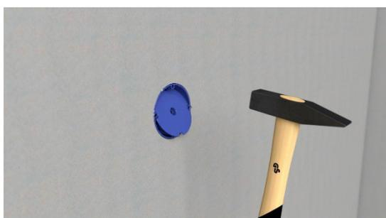
Open the lid with a hammer blow. There is no need to search for the box after plastering. In addition, there is no need for rework such as fitting leveling rings and filling the damaged plaster.
