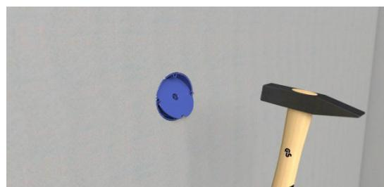
Break out the cover with a hammer and install the built-in appliance/socket.
