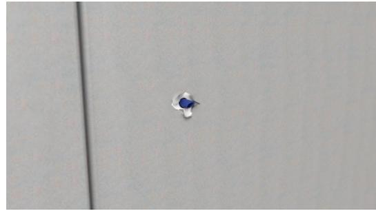
Press on the plasterboard until the spike penetrates.
