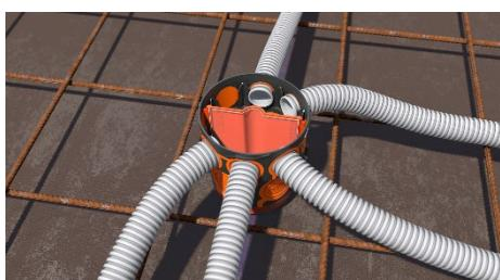
Insert the divider into the box before concreting.
