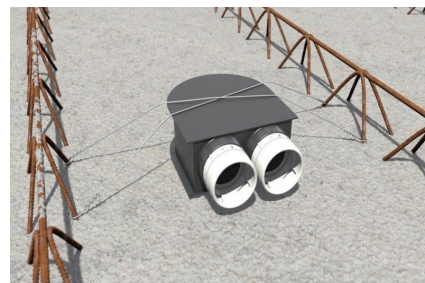
Insert the ventilation distributor into the ventilation sleeve. The ventilation distributor can be aligned by 360 degrees. Fix the distributor to the reinforcement with wire.
