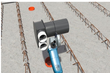
Shorten ventilation manifold to suitable length.
