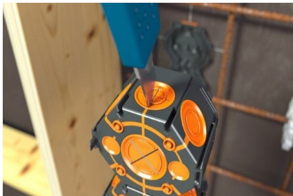
Open the diaphragm with a cutter knife.
