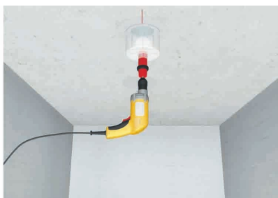
A can drill is used to drill out the individual opening...
