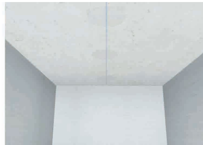
Mark alignment line, inaccuracies can now be corrected.
