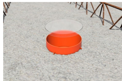
Remove the protective cover of the ventilation sleeve.
