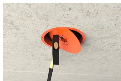
60 mm Remove magnet and open lid with a hammer blow.
